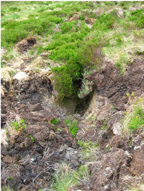
Figure 1. Poorly installed turf block which also caused extensive damaged to surrounding area.
